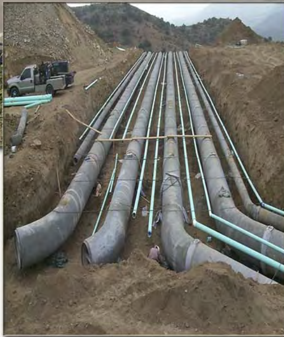
Pipes feeding the 640-1 and 640-2 Reservoirs
