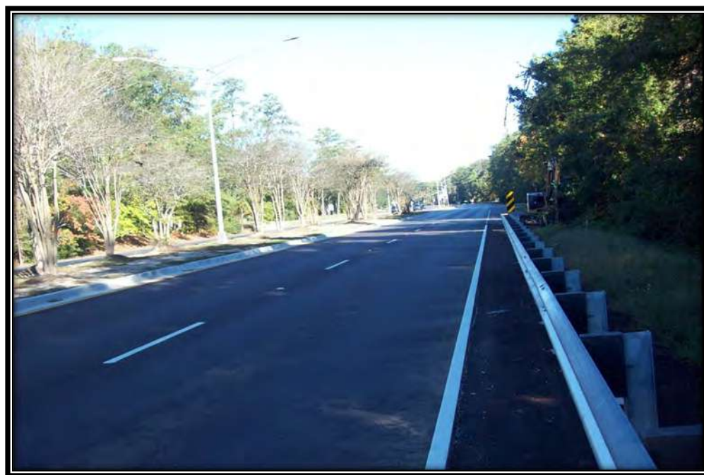
Figure 101 – New Overlay at Chinchuba Bridge West Approach
