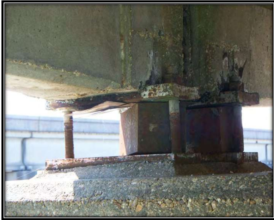
Figure 15 - Rocker Bearing Walking Out (SB Bridge)
