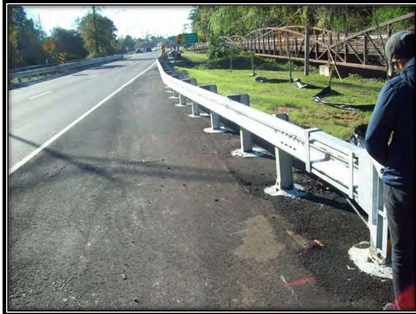
Figure 102 – New Guardrail at Chinchuba Bridge East Approach
