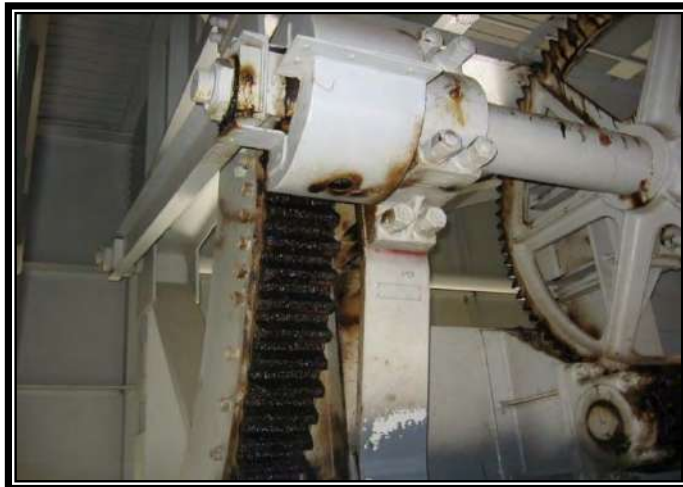
Figure 48 – Trunnion Rack, Bearing, Link Shaft and Spur Gear
