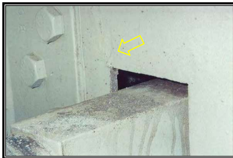
Figure 40 – Repaired Crack in Sidewalk Bracket Web
