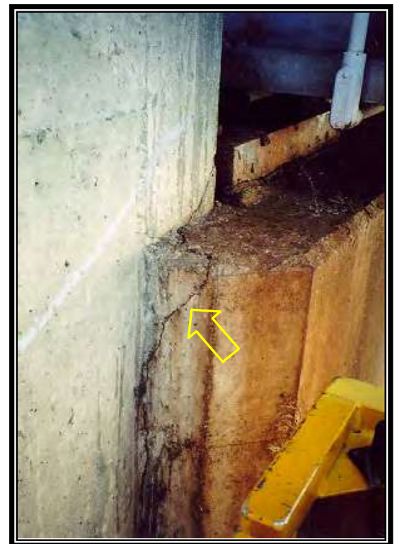
Figure 44 – Crack in Pier
