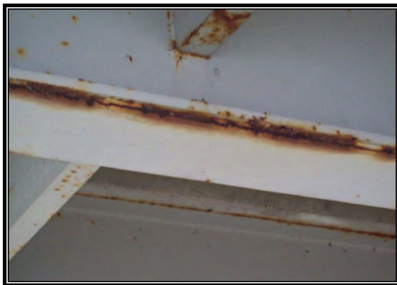
Figure 42 - Paint Deterioration at the Bascule Bridge
