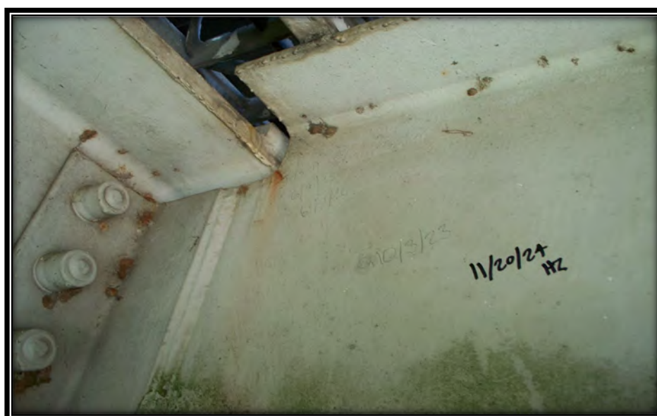
Figure 34 - Stringer Web -- With Inspection Notes
