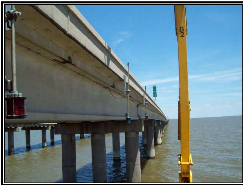
Figure 71 – Typical Navigation Light at North, Center and South Humps
