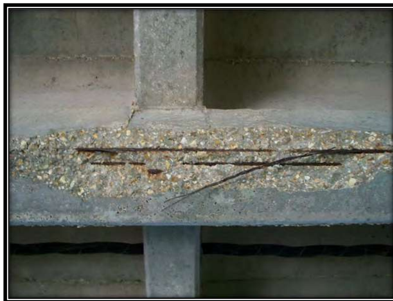
Figure 9 - Flange Loss with Exposed Prestressing Steel Tendons – Southbound
