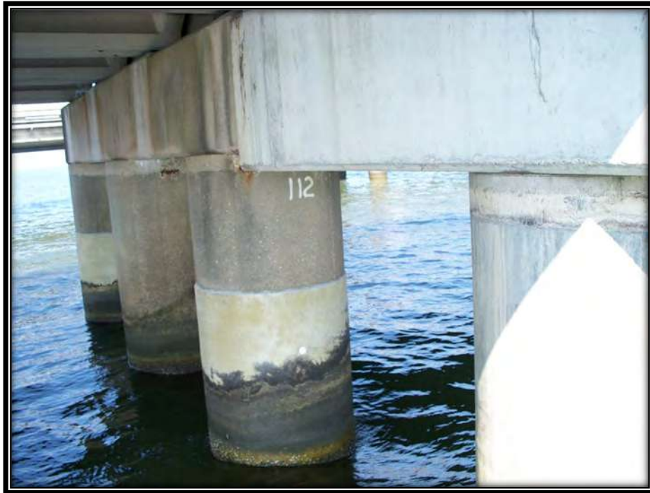
Figure 24 - Pile Encapsulation
