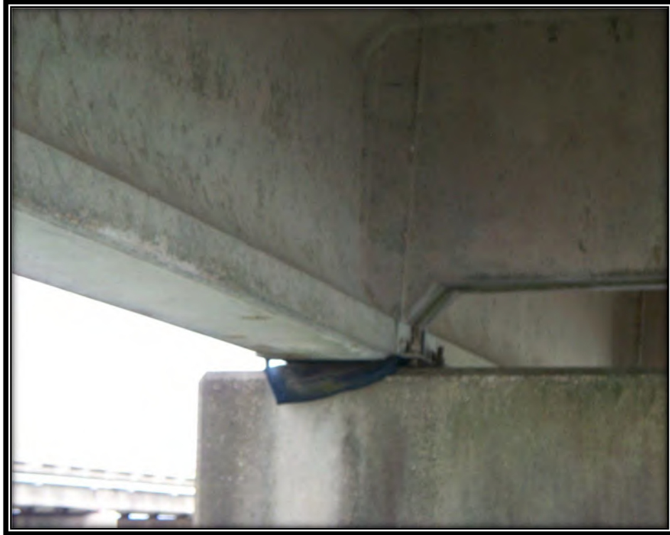
Figure 13 - Slipping Neoprene Bearing Pad (NB Bridge)
