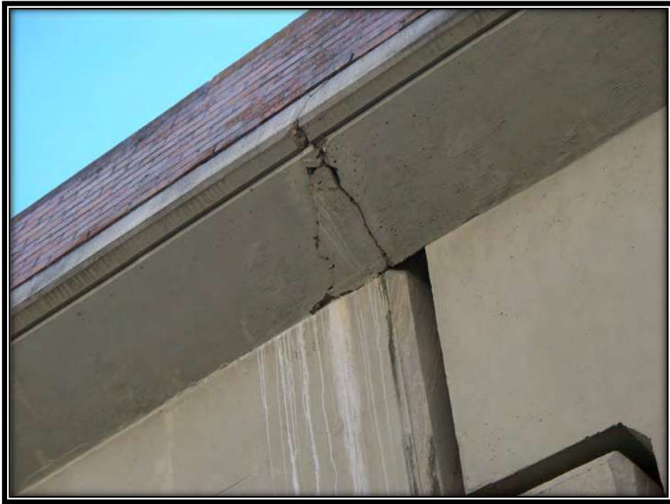
Figure 97 - Crack at Bent, NB Main Monroe Street Overpass
