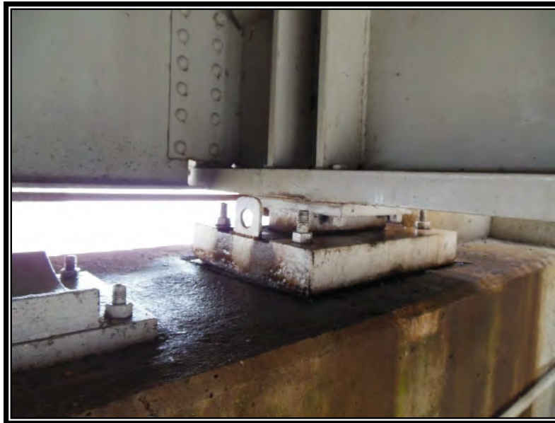
Figure 41 – Typical Live Load Bearing
