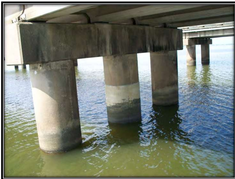
Figure 25 - Pile Encapsulation
