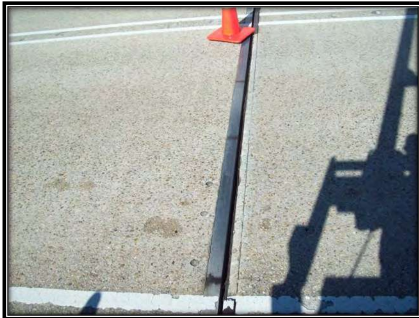
Figure 5 - Span 1000 End Dam Removed South End (NB)
