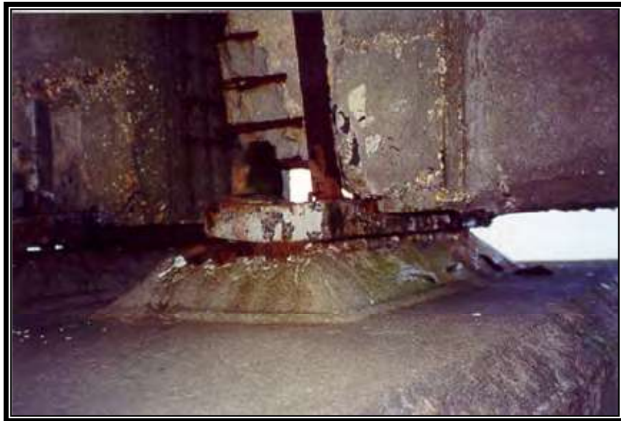
Figure 18 – Damaged Bearing Bent 1496 on SB Bridge (Prior to Repair)
