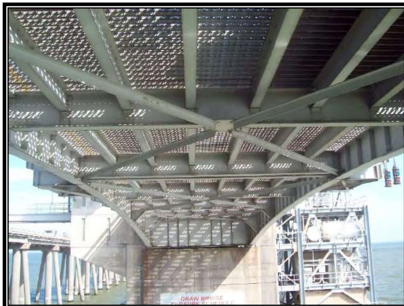
Figure 32 – Main Girders, Floor-Beams and Stringers
