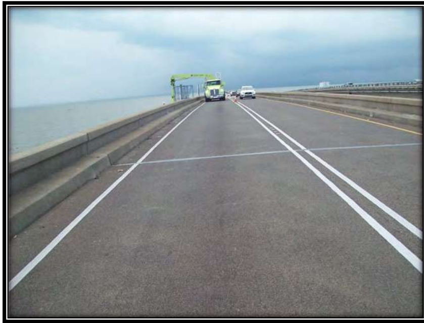
Figure 4 –Epoxy Overlay at the South Channel
