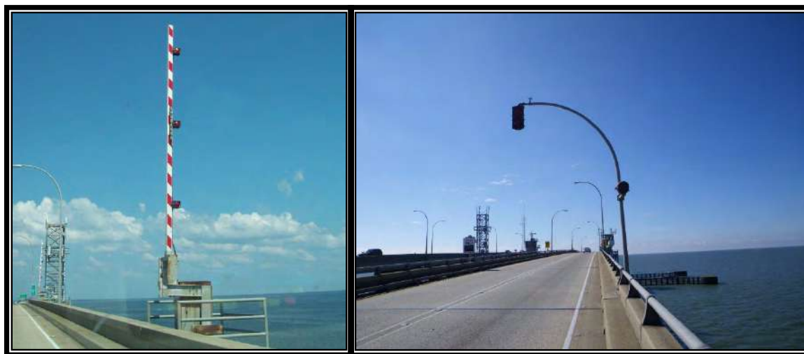
Figure 56 – Traffic Gate and Traffic Signal
