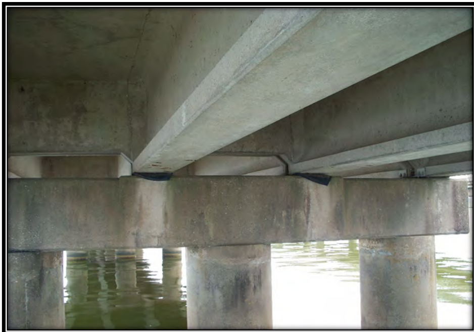
Figure 14 - Slipping Neoprene Bearing Pad (NB Bridge)
