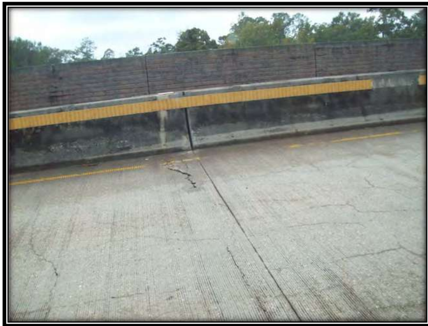
Figure 96 – Cracks on Bridge Deck, NB Monroe Street Main
