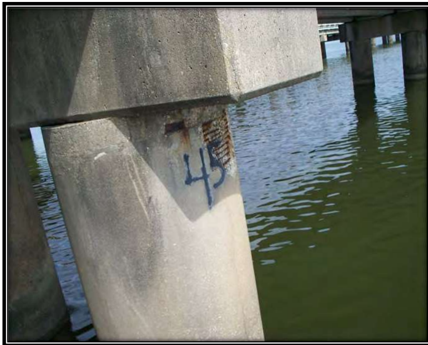
Figure 23 - Spalling on Pile
