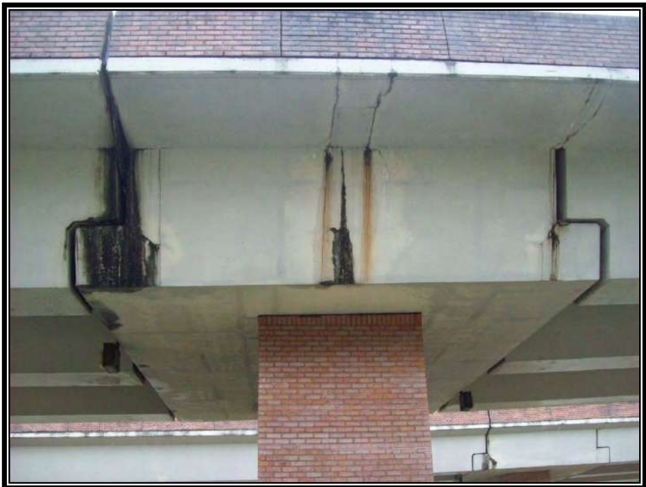
Figure 98 - Spalling on Bent, Monroe Street Overpass
