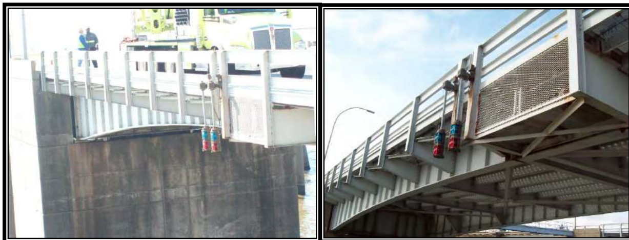
Figure 55 – Navigation Lighting
