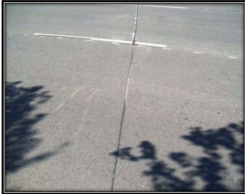
Figure 99 – Joints Repaired on NB Chinchuba Bridge
