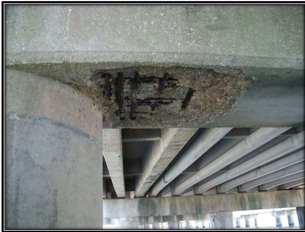
Figure 21 – Spall on Southbound Bent Cap
