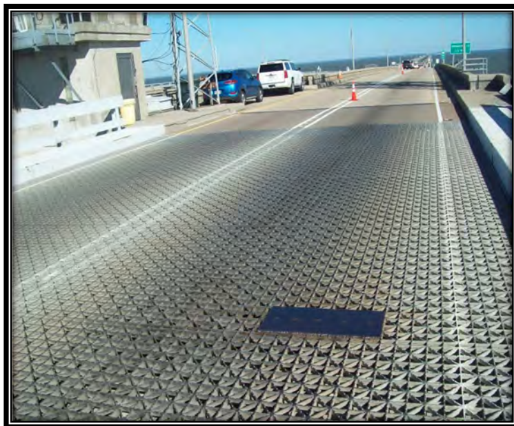
Figure 30 - Grid Deck on NB Bridge with Patch Plate
