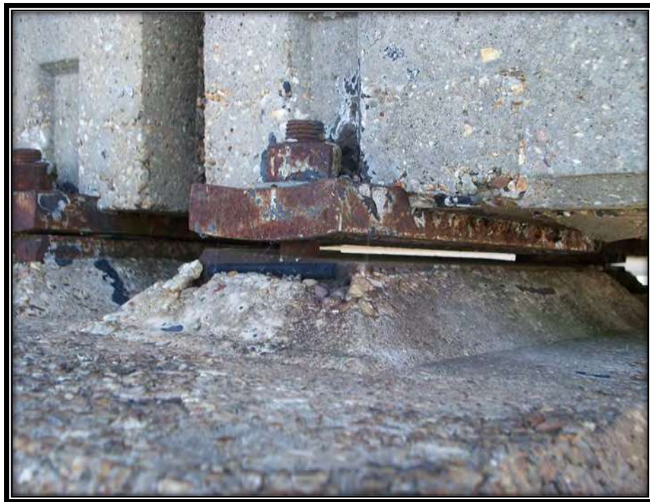
Figure 16 – Corrosion of Bearing Plates at Span 752 North End (SB Bridge)
