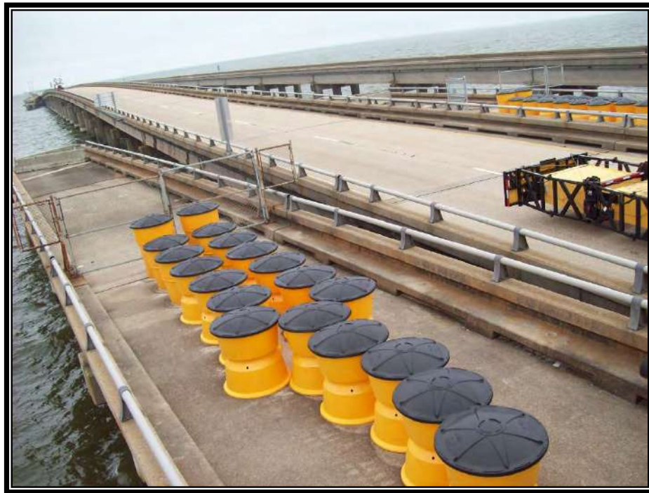
Figure 78 – New Impact Attenuator on Stub Ramps
