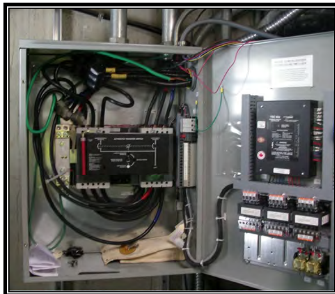
Figure 52 - Automatic Transfer Switch
