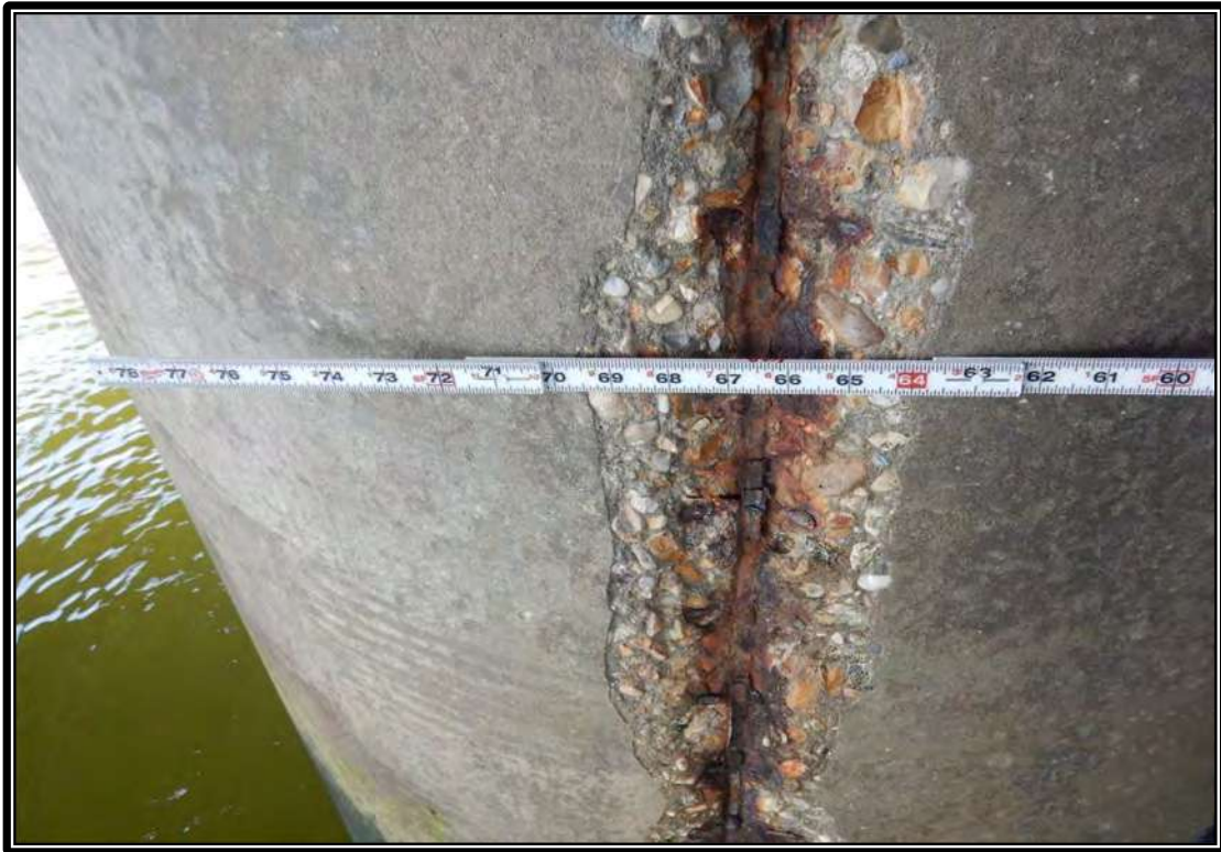
Figure 29 – Bent 657, Pile C – Spall above Water Exposed and Severely Corroded Longitudinal No. 3 Steel
