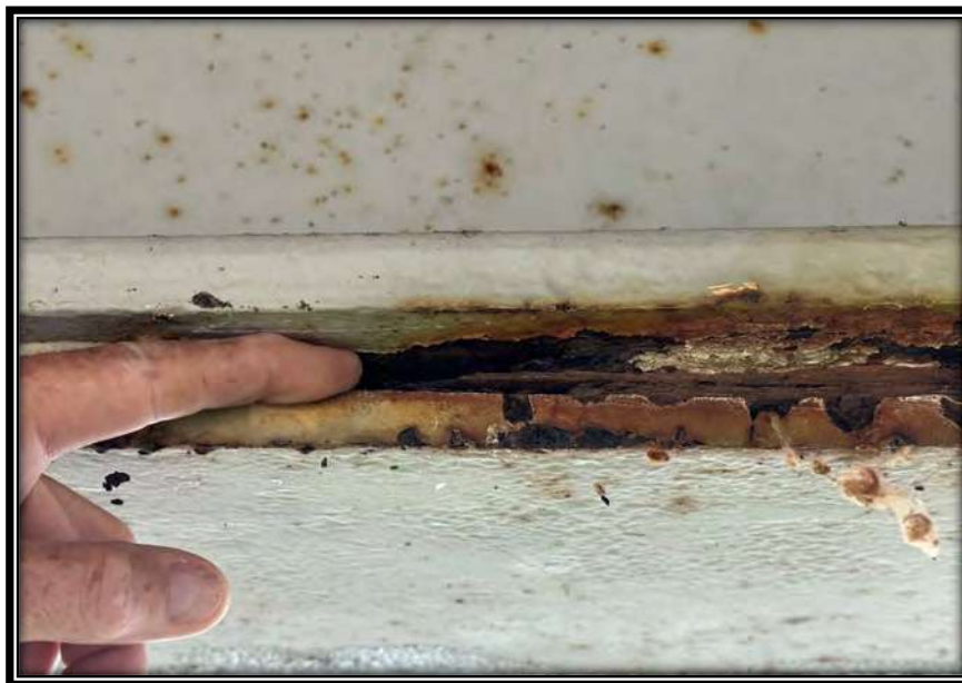
Figure 64 – Span 1876 Weld Crack on South Hump Steel Girder
