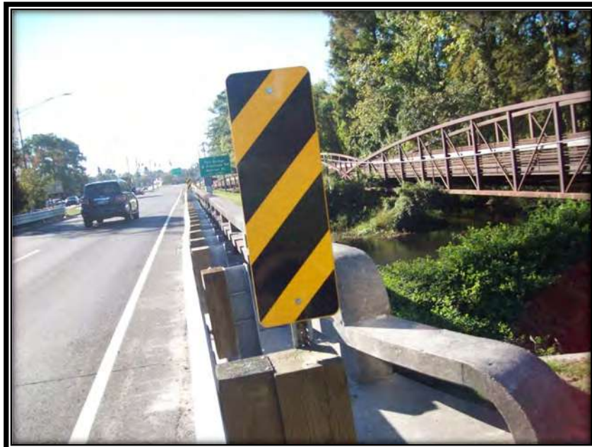
Figure 103 – New Hazard Marker at Chinchuba Bridge East Approach
