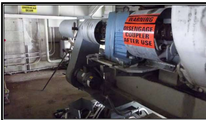
Figure 53 – Auxiliary Span Motor
