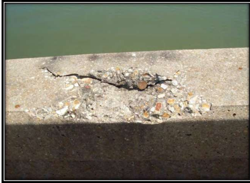
Figure 1 – Typical Damage to Barrier Rail from Lightning Strike
