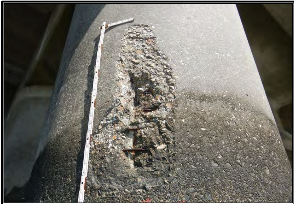
Figure 28 – Bent 623, Pile C – Spall above Water with one Exposed and Broken Steel Tendon
