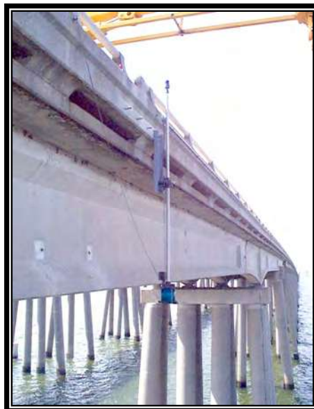
Figure 70 – Navigation Light at South Channel
