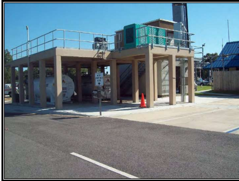
Figure 114 – Emergency Generator and Fueling Station at North Toll Plaza
