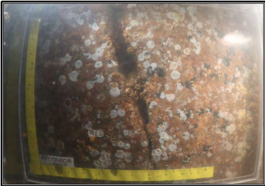
Figure 27 – Bent 755, Pile A – One of Two Longitudinal Cracks Below Water up to 5 Feet High by 1 Inch Wide
