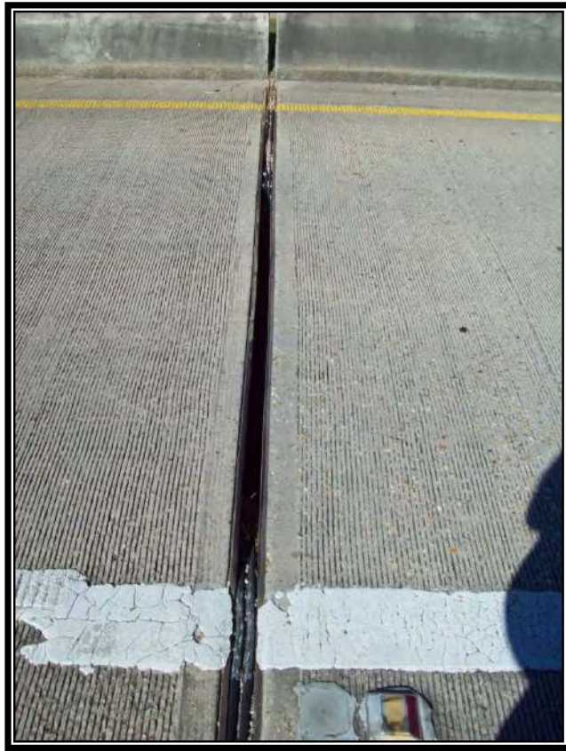
Figure 95 – Damaged Expansion Joint Seal
