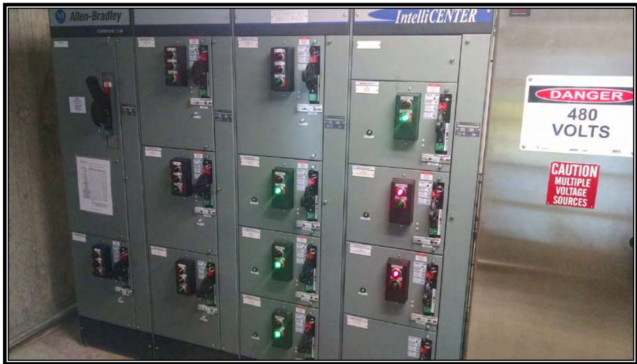
Figure 61 – Motor Control Center
