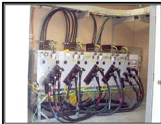
Figure 51 – Typical 5 Position Load Break Switch
