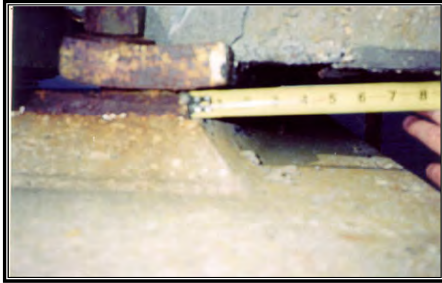
Figure 19 – Movement of Bent 1496 on SB Bridge (Prior to Repair)
