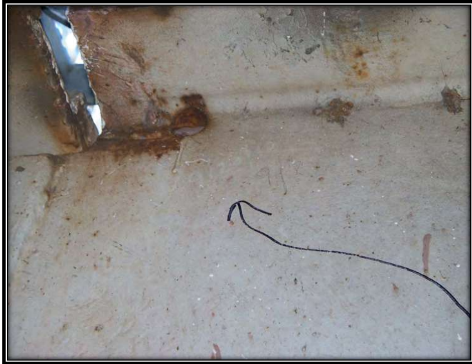
Figure 35 - Repaired Stringer Bracket - Crack Stopped by Drilling Hole
