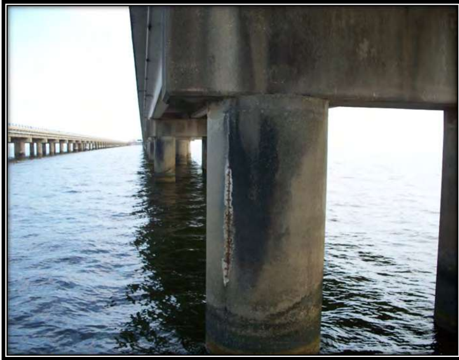
Figure 22 – Spalling on Pile
