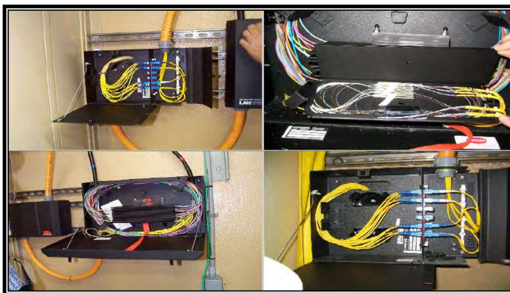
Figure 73 – Typical Fiber Optic Termination Housing and Splice Enclosure
