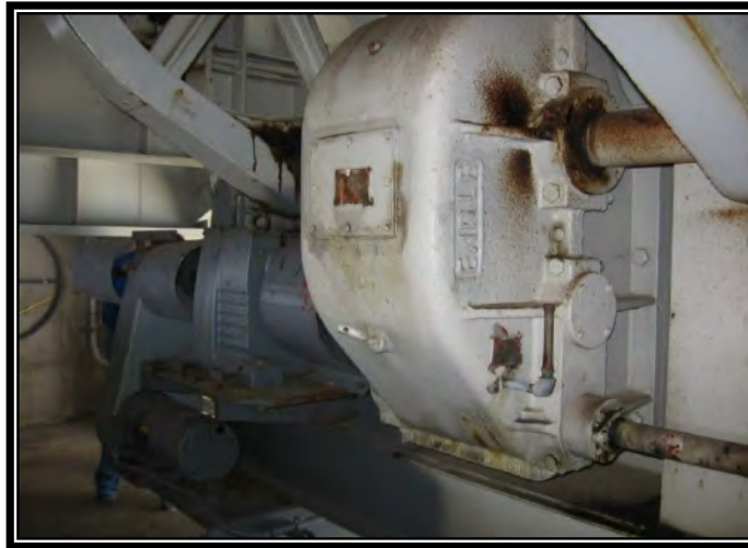
Figure 47 – Earle Gear Reducer and Auxiliary Span Motor
