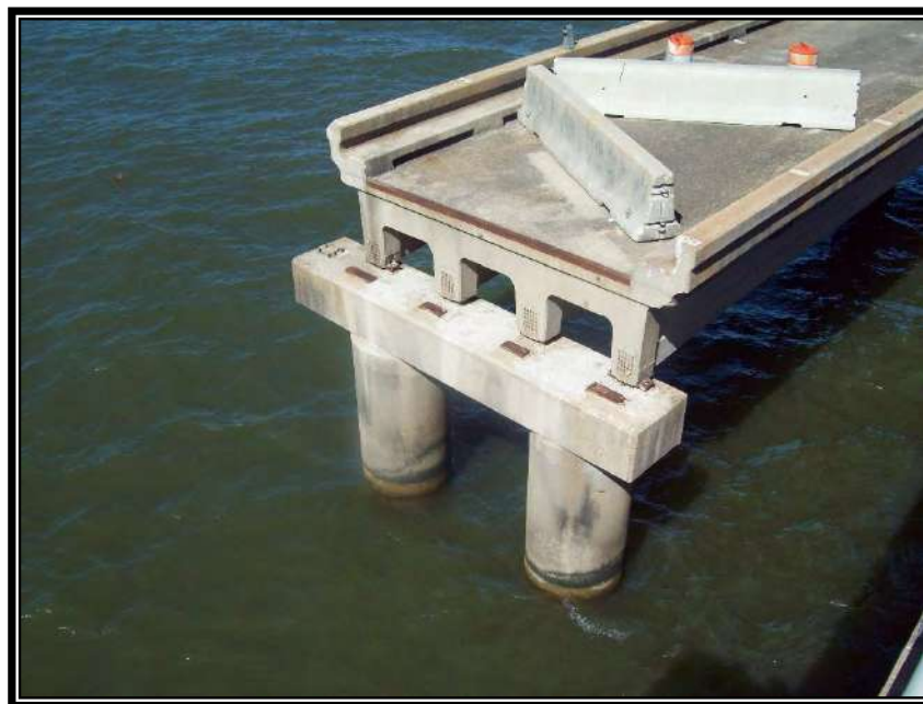
Figure 75 – Typical Concrete Barrier Placement on 9-Mile Turnaround Ramps
