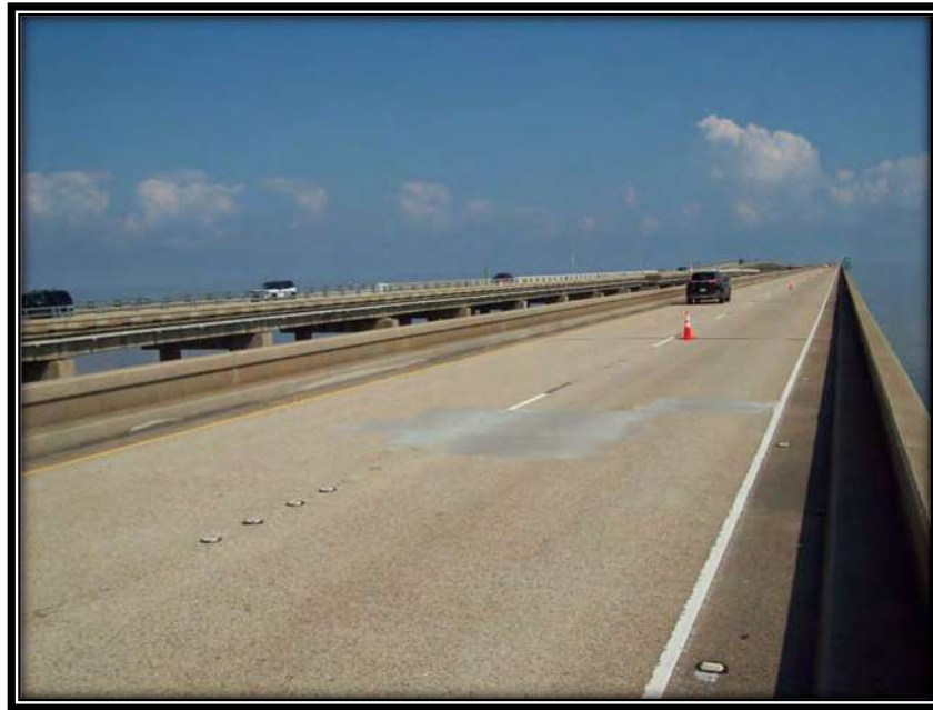
Figure 3 – Typical Bridge Deck Patch (Span 549 NB)
