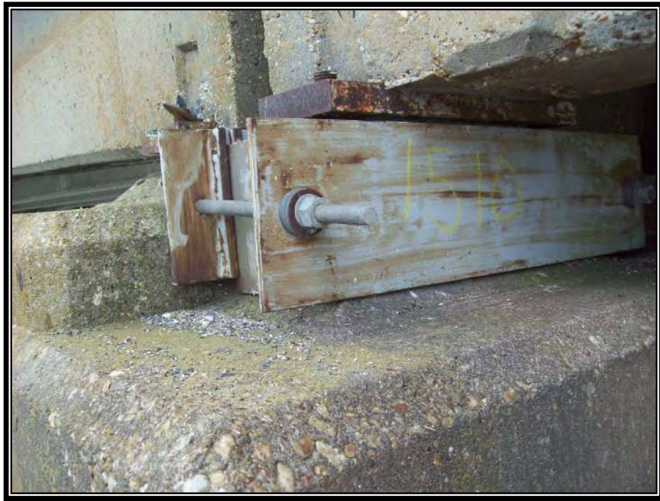
Figure 17 - Repair of Bent 1510 (SB Bridge)
