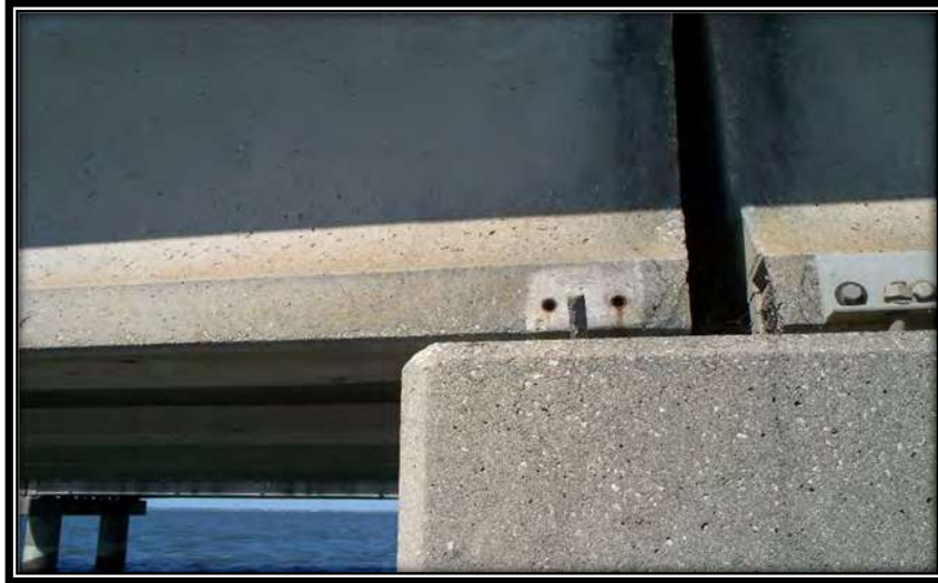
Figure 10 - Bearing Anchor Missing at Span 98 North End (NB)
