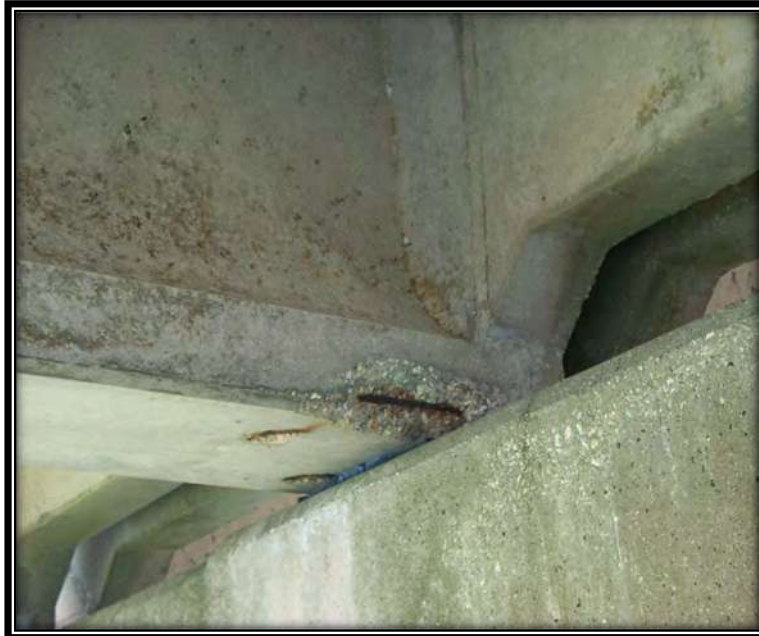
Figure 6 – Small Spall (>1 sq. ft.), Prestressing Steel Tendon Exposed
