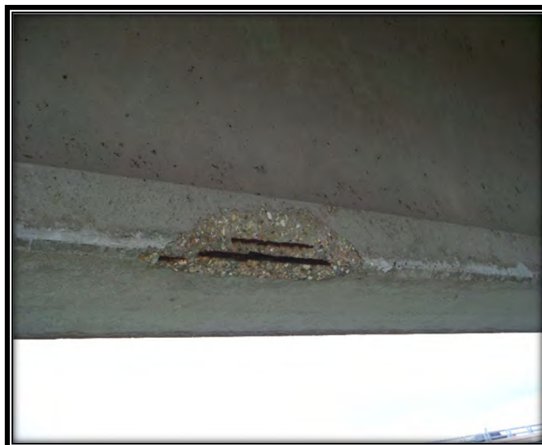
Figure 7 – Medium Spall (Between 1 and 3 sq. ft.) - Exposed Steel Prestressing Tendons
