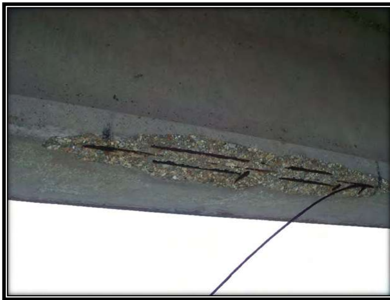
Figure 8 – Large Spall (< 3 sq. ft.) with Broken Prestressing Steel Tendons
