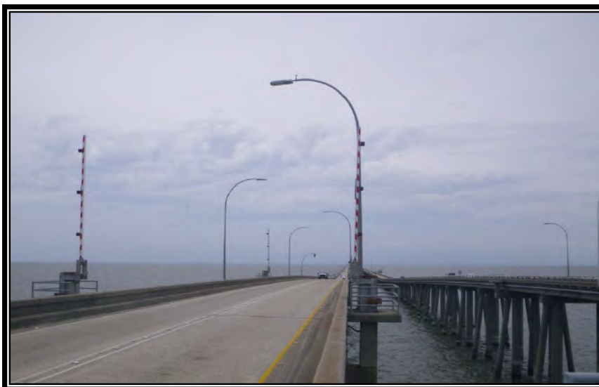
Figure 54 - Roadway Lighting and Traffic Gates
