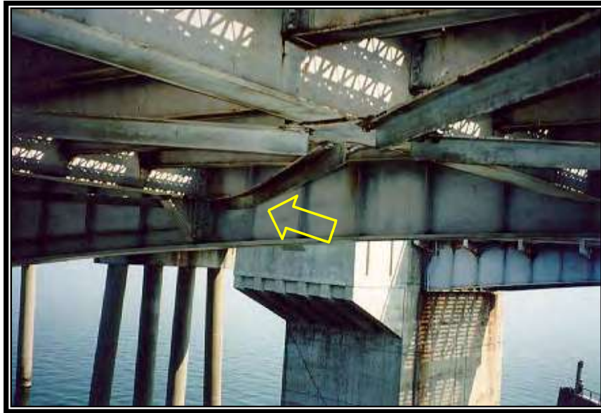
Figure 37 - Sagging Lateral Bracing
