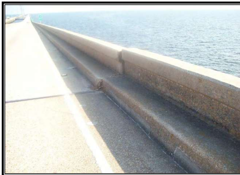
Figure 11 – Misalignment of Bridge Rail Indicating Lateral Shift of Span (500A/500B Northbound)
