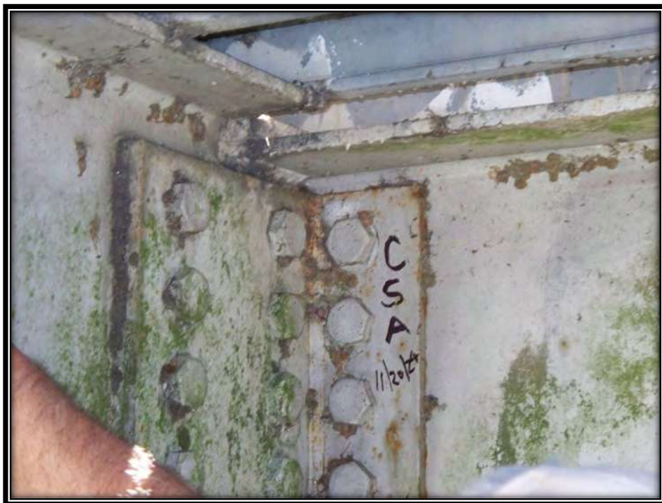
Figure 36 – Repair of Cracked Stringer Web
