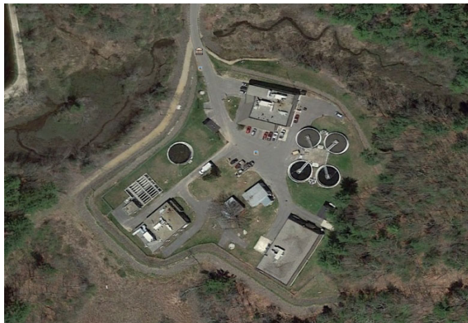
Kennebunk Water District's Treatment Facilities
