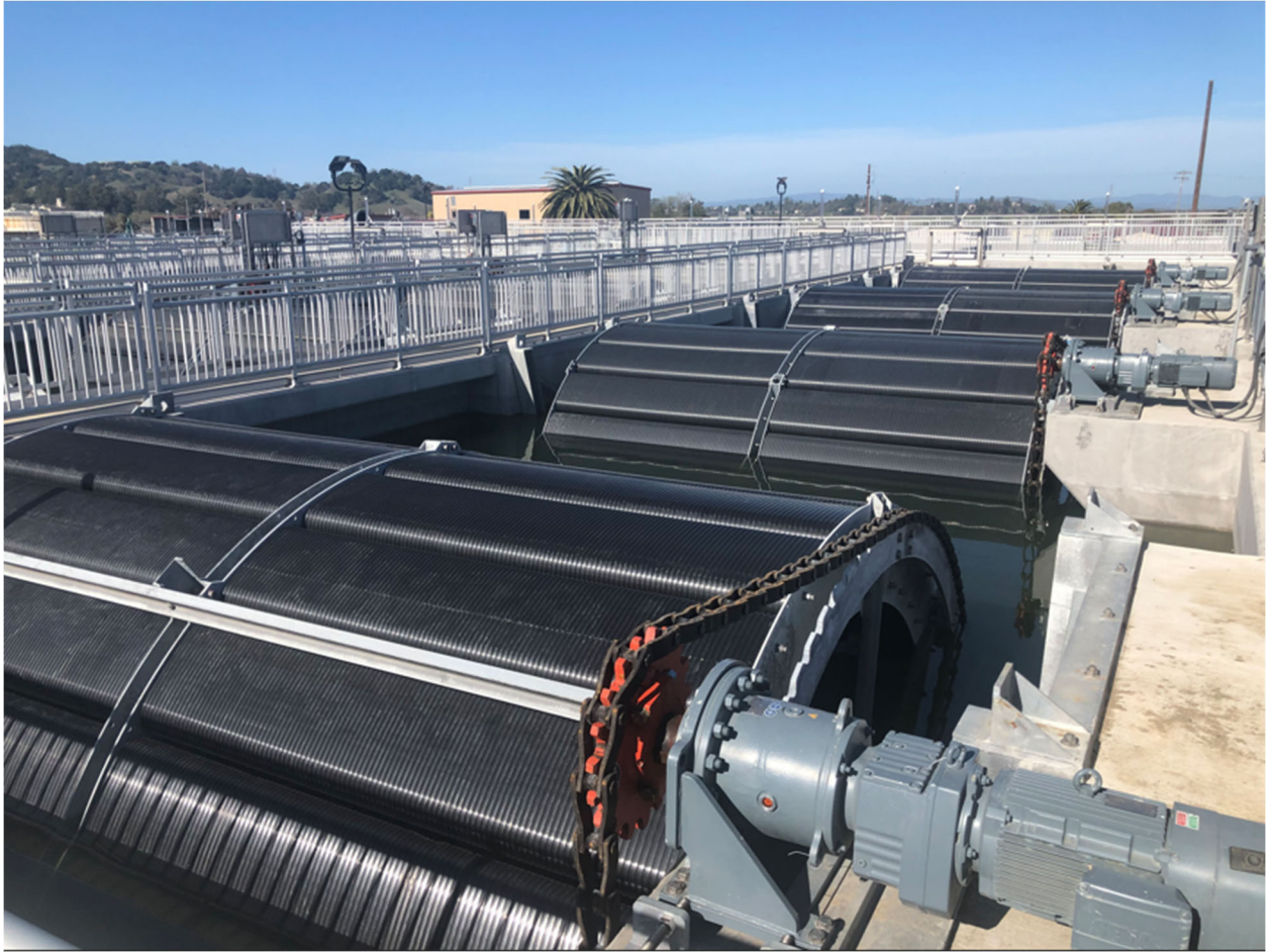
Biowheel aeration system
